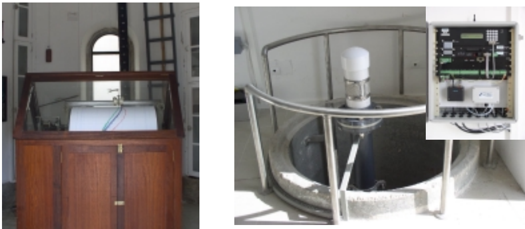
Figure 3 – Cascais tide gauges. Left: floating, right: acoustic.
